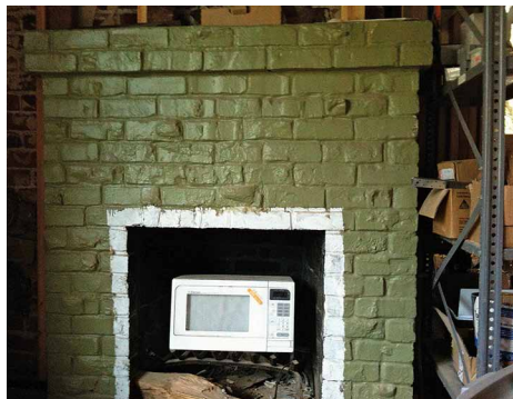
With multiple layers of paint, a clinker-brick fireplace in a 1905 house was too far gone to save, so designer Michelle Nelson created a new covering.
